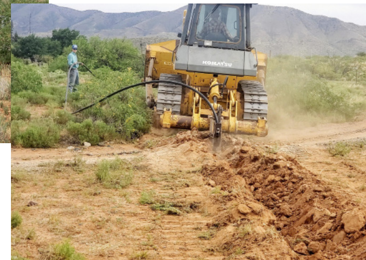
Adding water pipeline on the ranch.
